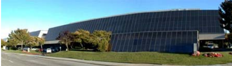
Yokowo America Corporation, Silicon Valley Office Complex
