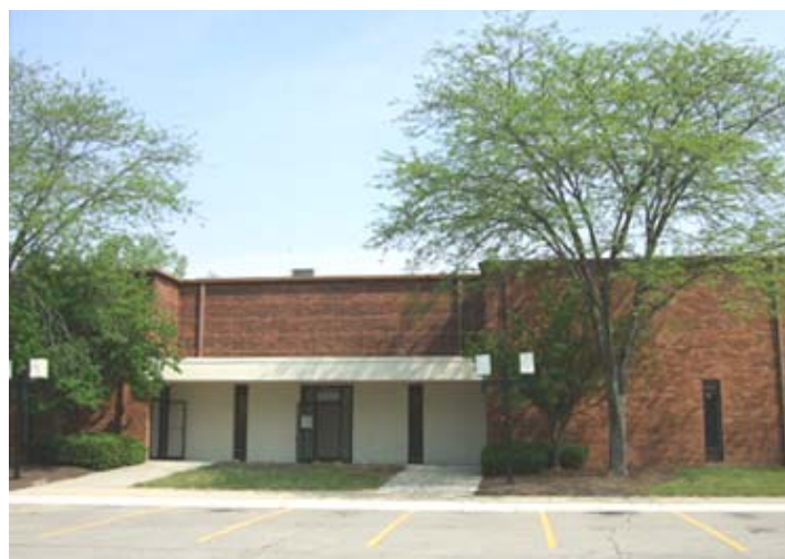
Yokowo Manufacturing of America LLC 新工場外観
